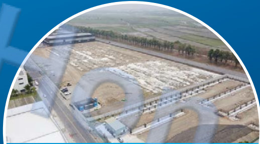
Kaohsiung HoFa Battery Center
